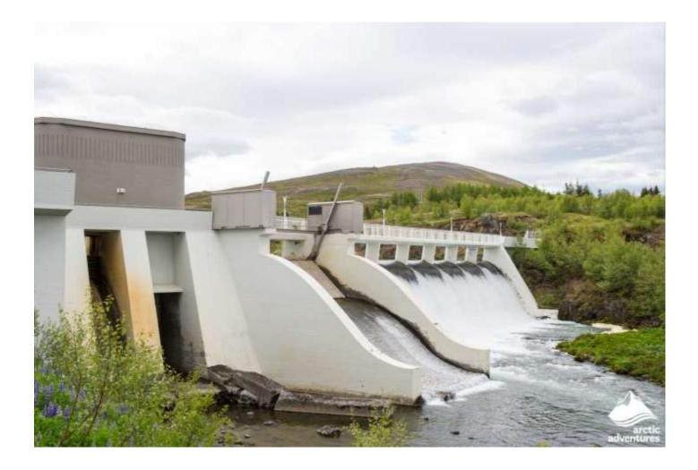
Hydroelectric plants consist of a dam and an engine room. The dam holds water, which is then gradually released through water turbines that generate electricity.
